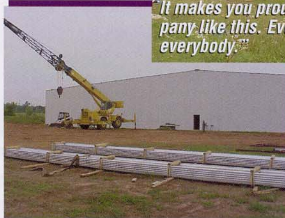
Rebuilding the facility.
